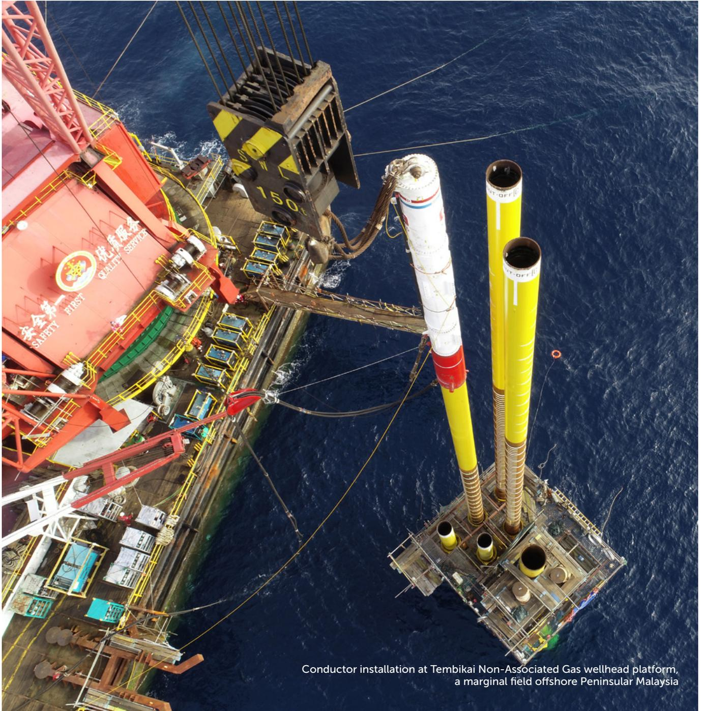
Conductor installation at Tembikai Non-Associated Gas wellhead platform, a marginal field offshore Peninsular Malaysia
